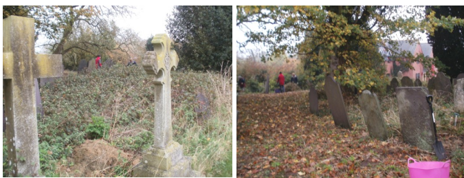
Work in progress in St Peter's Churchyard
